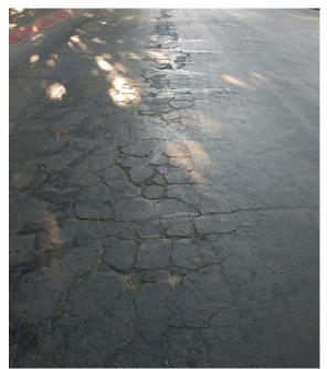
Figure 12: Fog sealed and striped road rated at 19 PCI (very Poor condition) located on F St in Los Banos.
