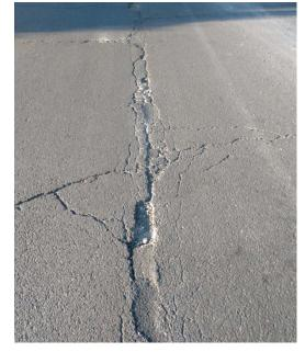
Figure 13: Fog sealed and striped road rated at 47 PCI (poor condition) located on 2<sup>nd</sup> Street in Los Banos.
