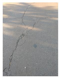
Figure 14: Fog sealed and striped road rated at 71 PCI (fair condition) located on 2<sup>nd</sup> Street in Los Banos.
